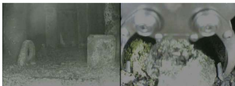
Fig. 2. Pollution in the hot gas chamber of the KS 150 reactor
