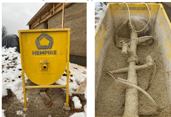
Fig. 3. External view of the mixer for in-situ hempcrete preparation
