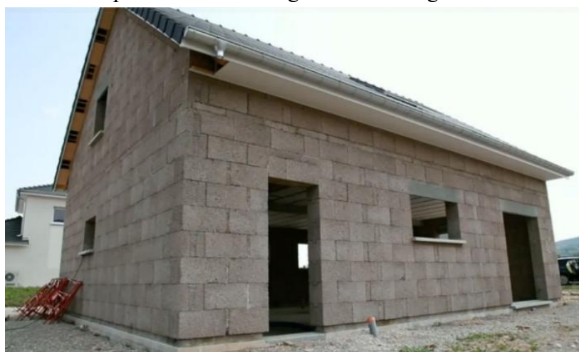
Fig. 4. Premanufactured hempcrete block building [12]
